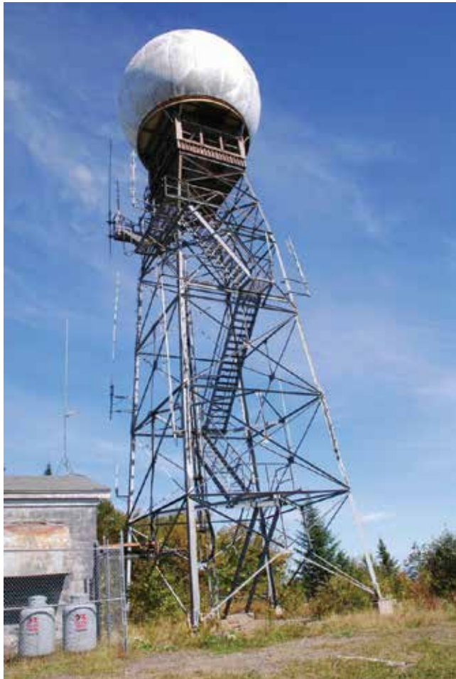
Pinetree Line Gap Filler Site. Photo courtesy of The Arctic Institute of North America.
